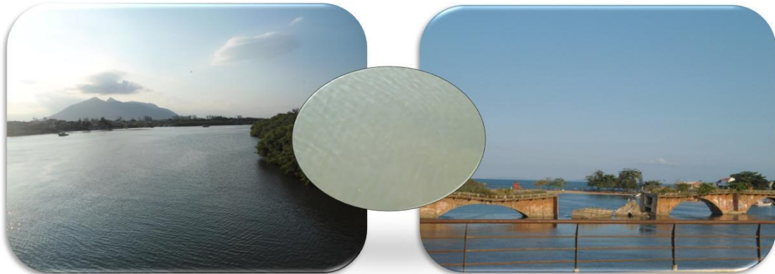
SJ #1 – Ponte RJ 106 – UTM 24 K 192007 7498245
