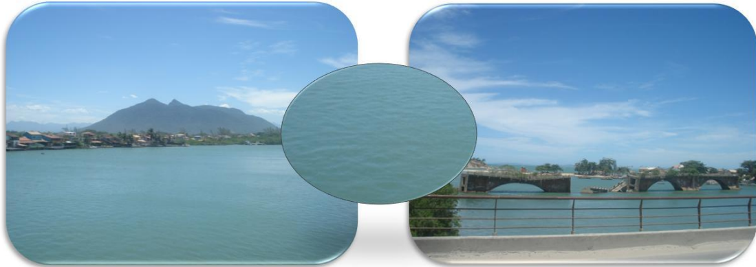
SJ #1 – Ponte RJ 106 – UTM 24 K 192007 7498245
