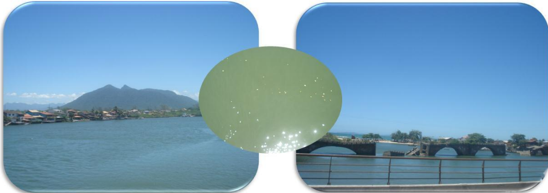
SJ #1 – Ponte RJ 106 – UTM 24 K 192007 7498245
